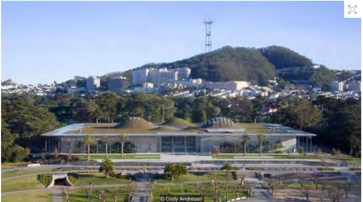
The intriguing design of the California Academy of Sciences is built to promote cooling air movement around the building (Credit: Cody Andresen)
