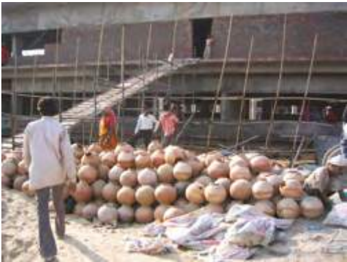
Matkas (earthen pots) sourced from local markets being assembled and installed on site
