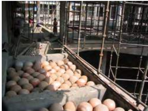
Matkas (earthen pots) sourced from local markets being assembled and installed on site
