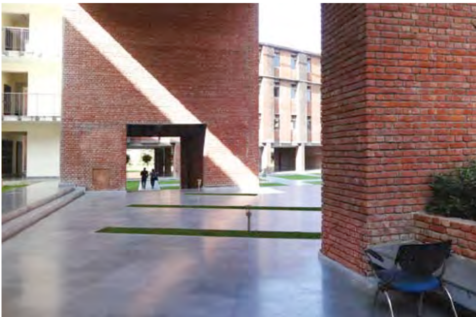
An orientation towards the north coupled with deep recessed windows provides maximum shade, adequate glare-free daylight and cross ventilation.
