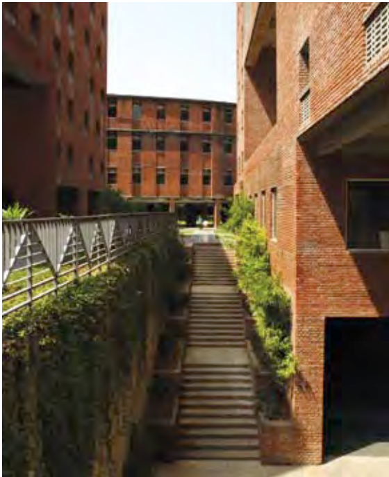
All movement has been aligned along one main street, with individual blocks looking into this primary circulation spine.
