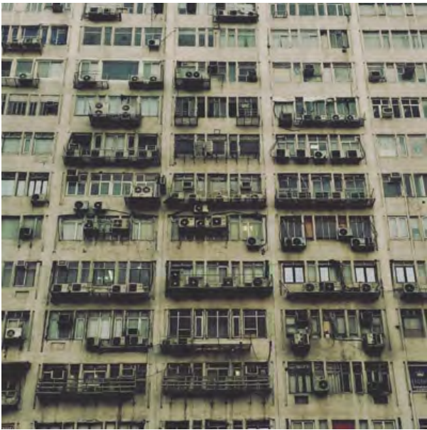
Air conditioners on a New Delhi high rise. (Photo credit: Milind Kaduskar)
