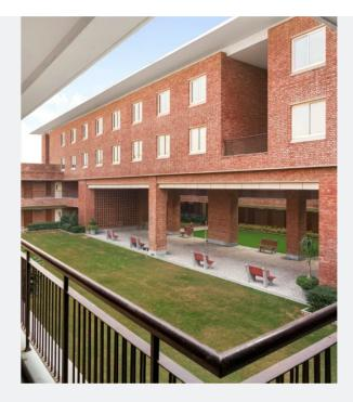
Using brick as a primary material was a no brainer. Undulations and perforations in the facade enable ventilation and shading in the corridors, while the overhangs prevent ingress of direct sunlight into the space, working concurrently to reduce heat gain. The design plays with different forms and levels of fenestrations, revealing interesting gaps, thus, reinventing the tradition of the jaali and jharokha (a type of overhanging enclosed balcony).
